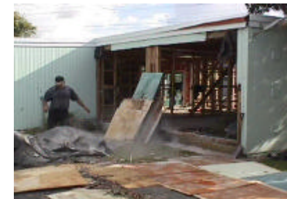
Demolition begins on new administration and student centre
